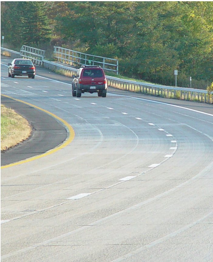
⚡ Completed diamond ground surface
