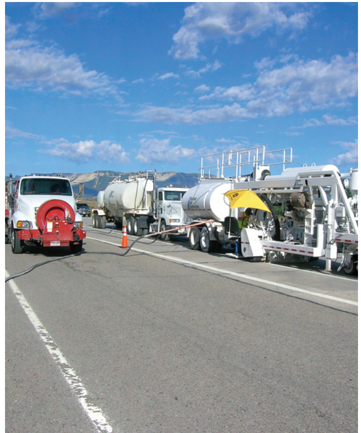
⚡ Diamond ground surface under construction
