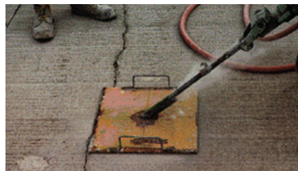
↗ 2. Simple drill rig that controls the starting location of drilling to ensure that hole intersects crack at about mid-depth.
