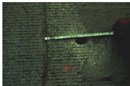
↗ 3. Checking hole location.
