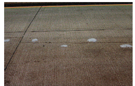
↗ 6. Completed cross-stitching on longitudinal joint.
